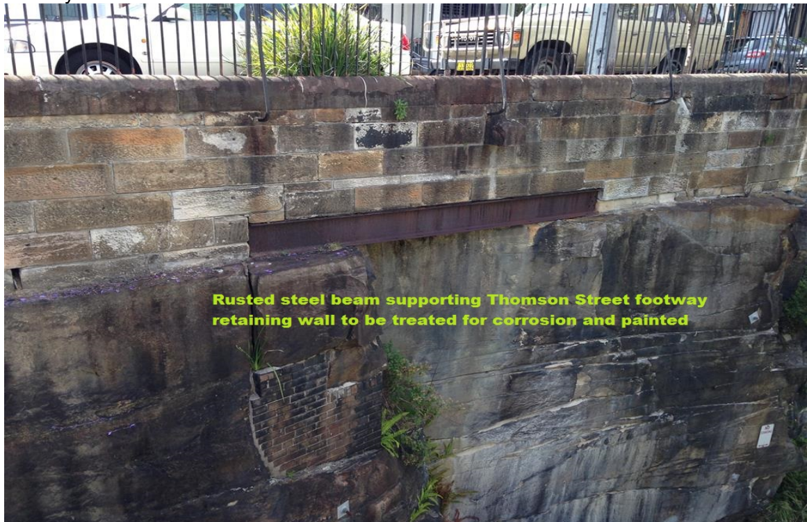
Photo 2 – Rusting beam supporting sandstone block wall that retains Thomson Street footway structure
